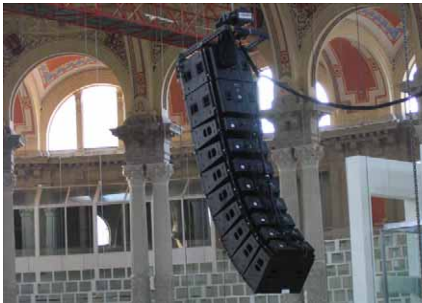
Figure 1.4: AX3210P array with overhead AX1118SP subs, a typical employment of vocal sound reinforcement in an indoor arena.
