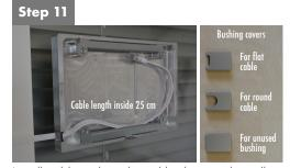
Install cable to the selected bushing and install appropriate cable cover. Cable length inside is 25 cm. Covers for flat and round cables as well as for unused bushings are delivered. Covers are fixed with adhesive tape.
