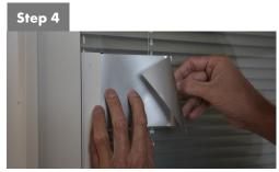
Use vertical ruler or level to adjust correct foil vertical position. Put foil on the wall with the protective film (not with adhesive part) to the ruler or level.
