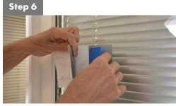
Partially remove the protective film and stick the rest of the foil using a squeegee.
