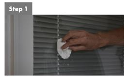
Degrease wall (typically glass) surface with alcohol and left it completely dry.
