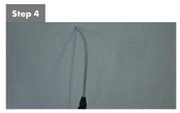
Install cable to appropriate position on the wall regarding restricted area described in previous step. Recommended cable length from the wall is 25 cm. Recommended height from floor to center of the panel is 1 500 mm.
