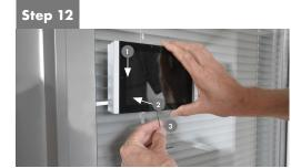
Connect Ethernet cable to the panel and put the panel on the back cover - 1, 2. Carefully tighten the fixing screw to fix panel on the back cover - 3.
