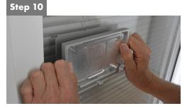
Degrease foil installed on the wall and left it completely dry. Remove protective film from the adhesive tape (installed on the rear side of the back cover) and carefully attach it on the foil installed on the wall
