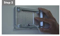
Install cable to the cable hole and put back cover on the wall. Position of back cover must be oriented as displayed above - cable bushings are left, right and bellow side oriented.
