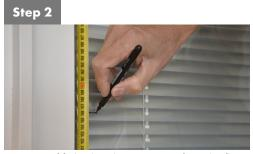
Sign top of foil in height 1 560 mm from the floor. It is for recommended height 1 500 mm from floor to center of the panel.
