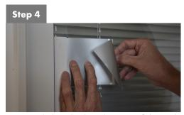
Use vertical ruler or level to adjust correct foil vertical position. Put foil on the wall with the protective film (not with adhesive part) to the ruler or level.
