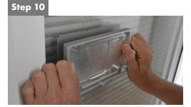
Degrease foil installed on the wall and left it completely dry. Remove protective film from the adhesive tape (installed on the rear side of the back cover) and carefully attach it on the foil installed on the wall
